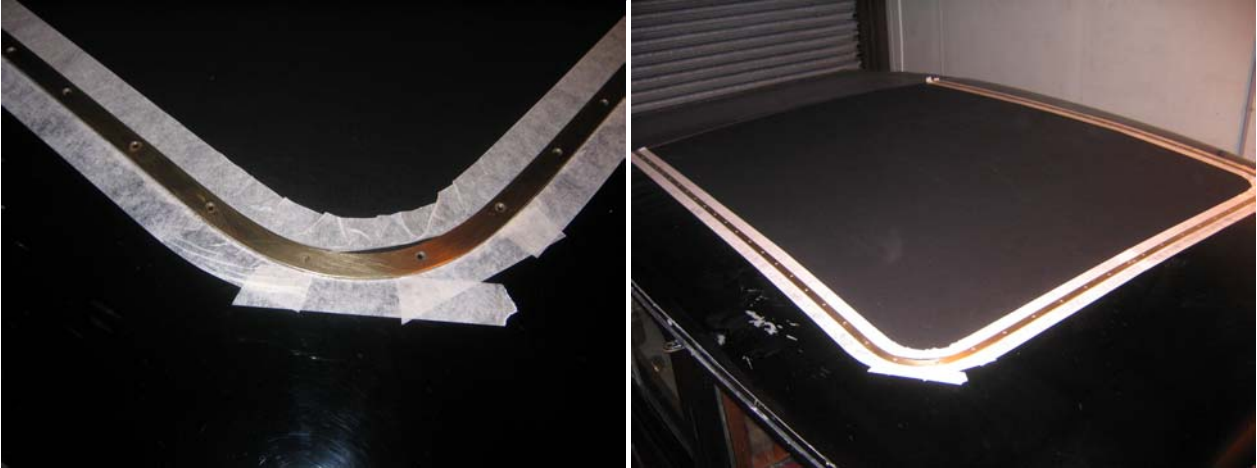
Taping up to create the final seal
